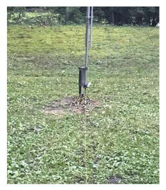
The visible radials were secured on top of the sod with lawn fabric staples and by this spring were completely covered.
