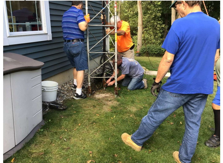
It's up. Get those bolts in place!
