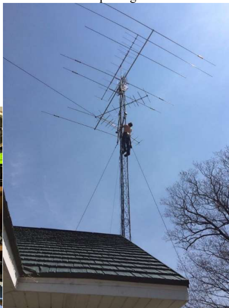
Dave's son repairing antenna
